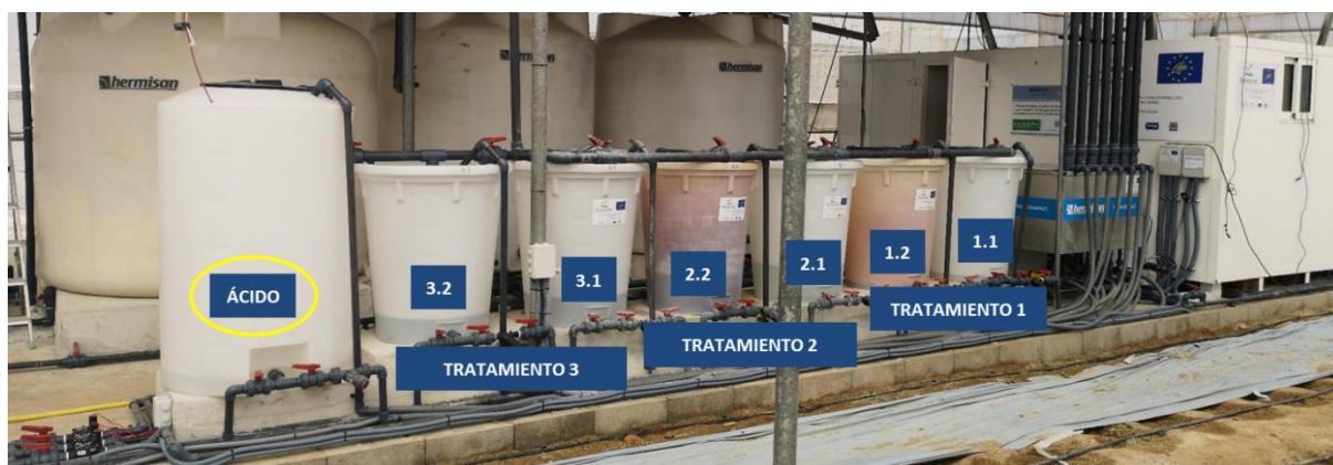
Fig. 6. Tanks per treatment in the irrigation head.
